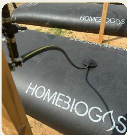
Gas pipe connection to the system
