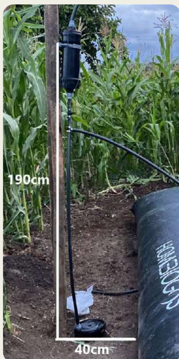
Connect the T-connector. It should be lower than the stove's table
