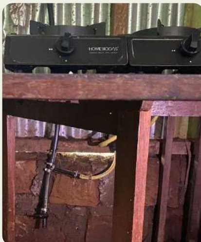
Connect the water trap. The position should be easily accessible to open it
