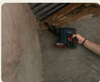
Drilling point in the kitchen wall
