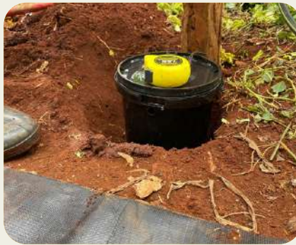
Place the pressure release mechanism into the hole.
